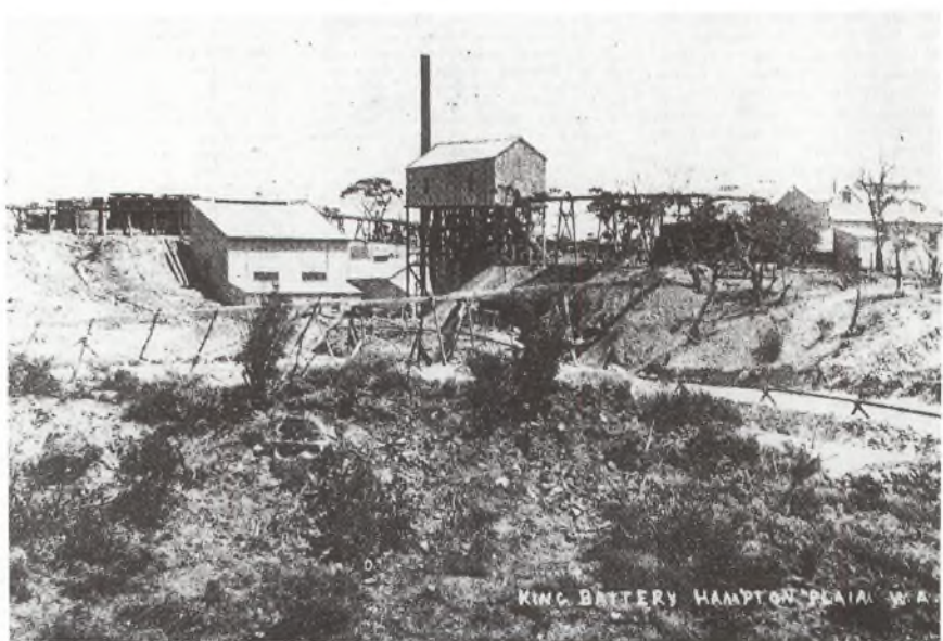
The completed King Battery, with a capacity to treat 100 tons per day. - 1902 The 20 head battery was fed by rail links to surrounding mines 8km SW (Merry Hampton) and 5km north (Hampton Boulder/Jubilee)
