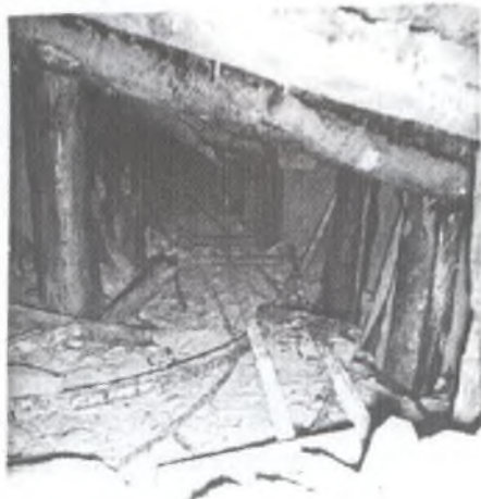
FIG. 29 LAKE VIEW LOGE TUNNEL ON N-7 LEVEL LOOKING NORTH FROM MAIN EAST CROSSCUT SHOWING EAST LEG SUGGESTED 2 FT WITH BLOCK MOVEMENT
