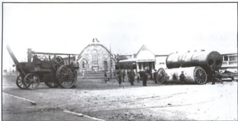
In 1911, the Kalgoorlie Brewery installed these large boilers (right) into their Porter Street premises, using the traction engine on the left to put them in place. The veranda posts of the Roads Board Chambers can be seen at left. Wesley St. Paul's church is visible in the background.
