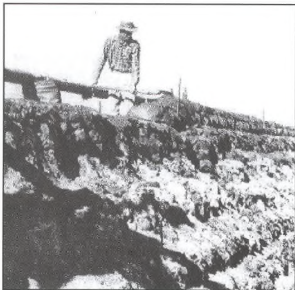
Shovelling up a lip of "tails mud" in the formation of "slime dump".
