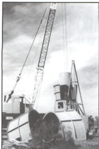
(above) A 20 tonne, 100 inch Axial flow mine exhaust fan supplied to Mt.Charlotte Gold Mine, 1967.
