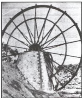
Tailings wheel as it remained in the mid 1950s. Note: relative size of the 3 people on the 60 foot wheel rim. The wheel was burned and destroyed by vandals several years after this photo was taken.
