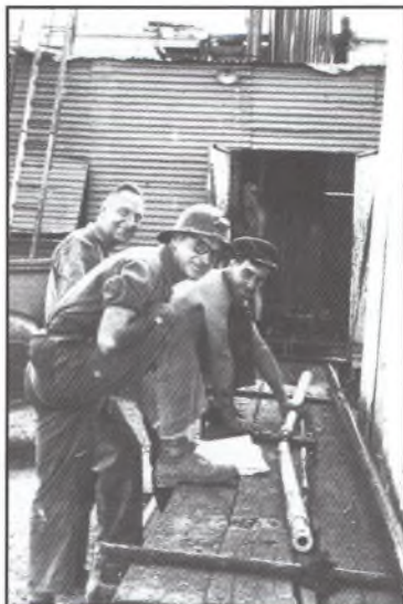
Gordon Buller, Les Grant & George Morrow examine the arc-cutting-device on hole SE7, beneath the angle headframe on Hannan's Lake, Circa 1960.
