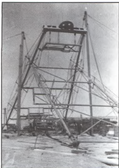
The angle headframe being erected for the first time. Hannan's Lake, mid 1950's.
