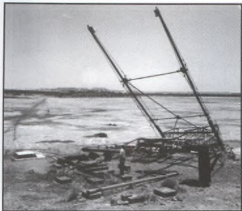
(right) Smashed head pulley that had pulled countless drill rods.
